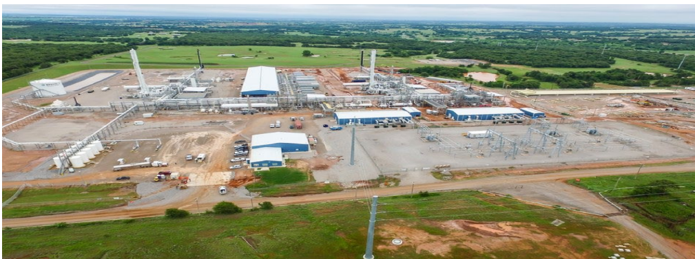
Process Photo no. 2 – Natural Gas Processing Facility
